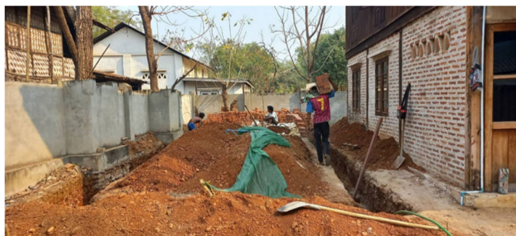
Construction of the store room begins...
